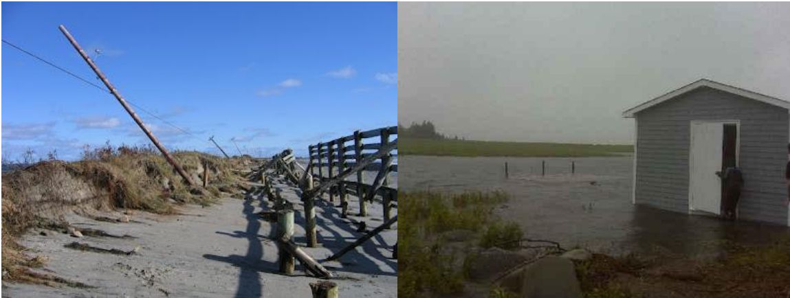
Figure 1:4 (a) Crescent Beach following Post-Tropical Storm Noel in 2007. Source: http://hurricane-noel-nova-scotia-damage.blogspot.ca/2007/11/photos-of-dammage-to-crescent-beach-and.html . (b) Damage at Petite Riviere caused by Hurricane Bill in 2009. Source: http://www.theweathernetwork.com/your_weather/details/786/1442612/bridgewater/hits/1#utmxd=EAAAACD_N29-7CmDyYe4sM7ENrk;utmxdpreview=0 .
