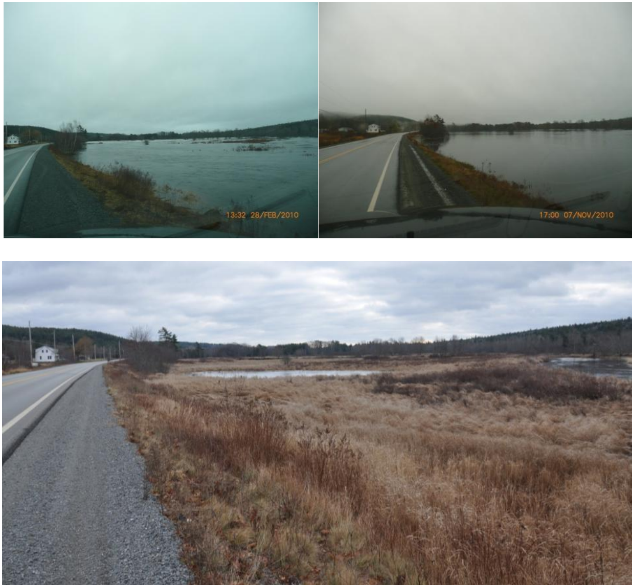
Figure 1:27 A section of Highway 10 near New Germany during flooding in February, 2010 (top left) and November, 2010 (top right); the bottom photo is from December, 2012 during non-flood conditions.
