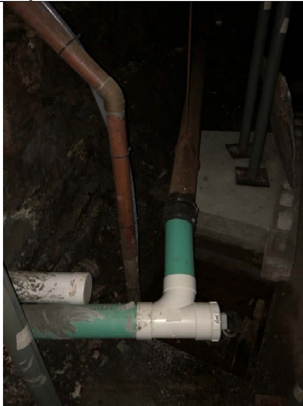
Photograph 2 – Wastewater Lateral to King Street Cross Connection Noted. Flush Test conducted to confirm Wastewater Connection.
