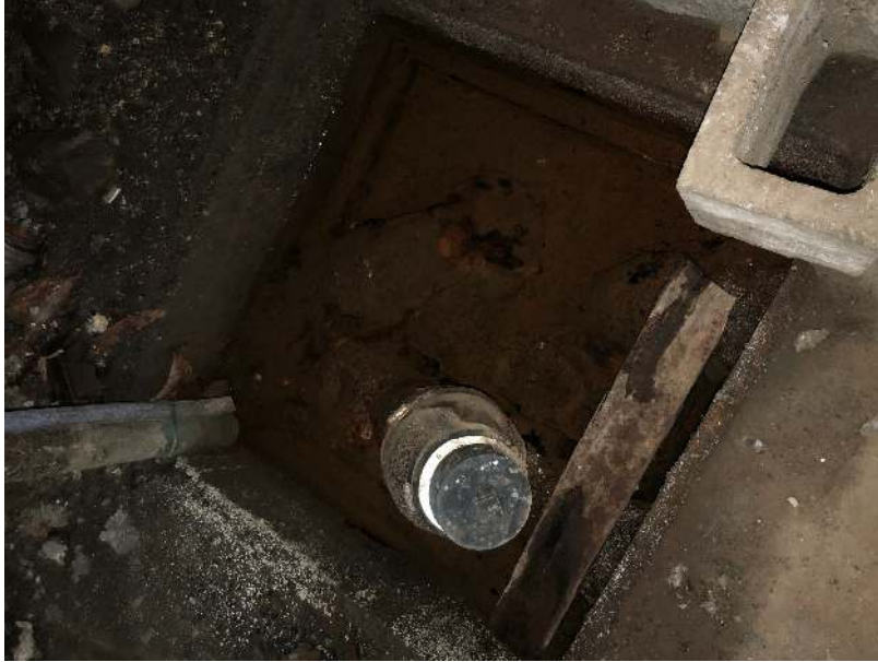
Photograph 1 – Existing Sump Pit.
